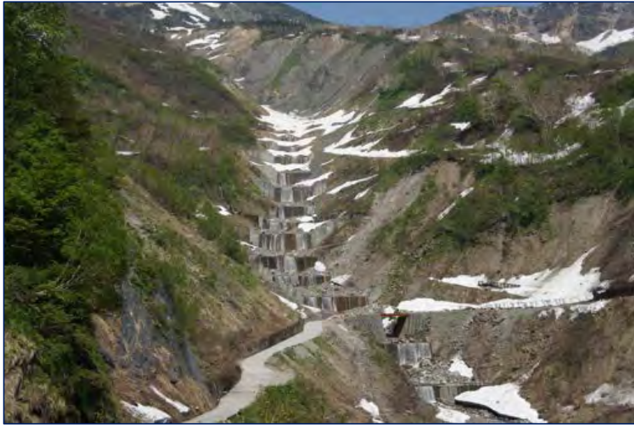
The upper Tedorigawa River Valley is heavily engineered by a series of check dams which inhibit the process of mass transport—a key characteristic of a the geomorphology of a dynamic river system
