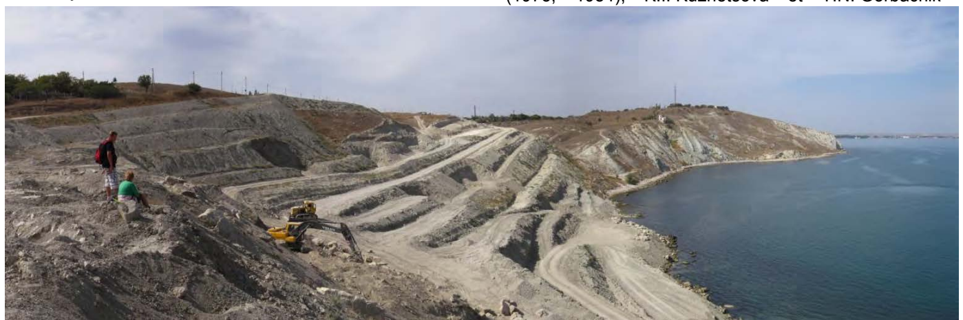
Fig. 2. The scale of excavation works is shown on sea conservation zone (photo Yu. Veklich)
