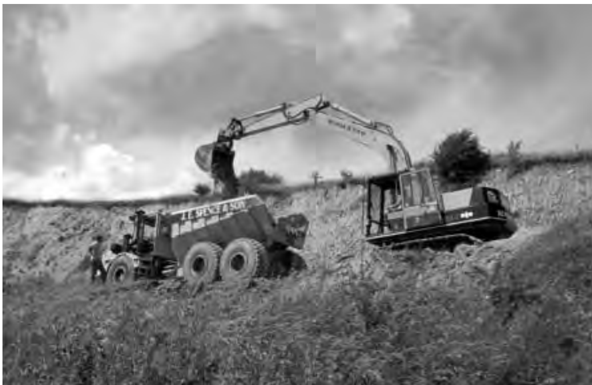
Clearance works underway at Welton-le-Wold (Photo John Arum)
