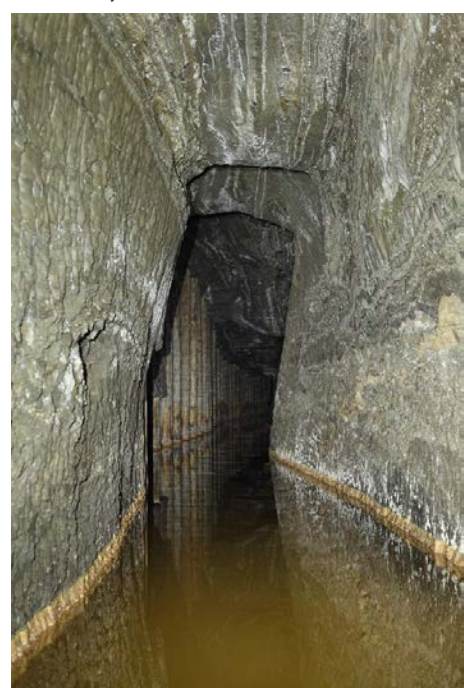
Figure 1 : Gallery partly filled with brine.
