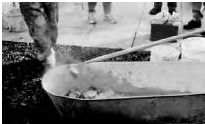
Demonstration of quicklime for use as mortar in restoration, by Scottish Lime. Photo: Sylvia Smith-Meyer
